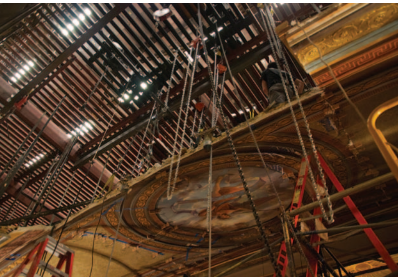
Ceiling piece with cartouche being put into place
