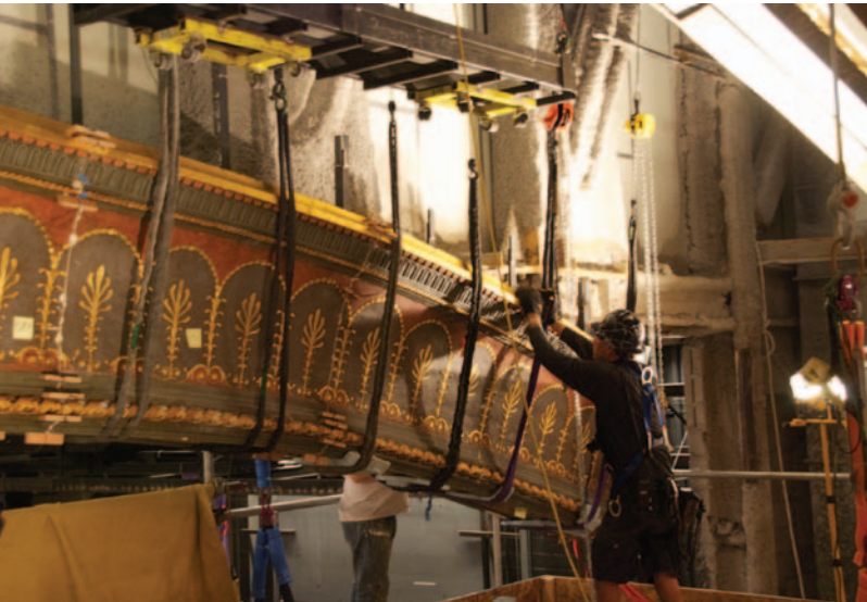
Riggers put the theatre proscenium back in place
