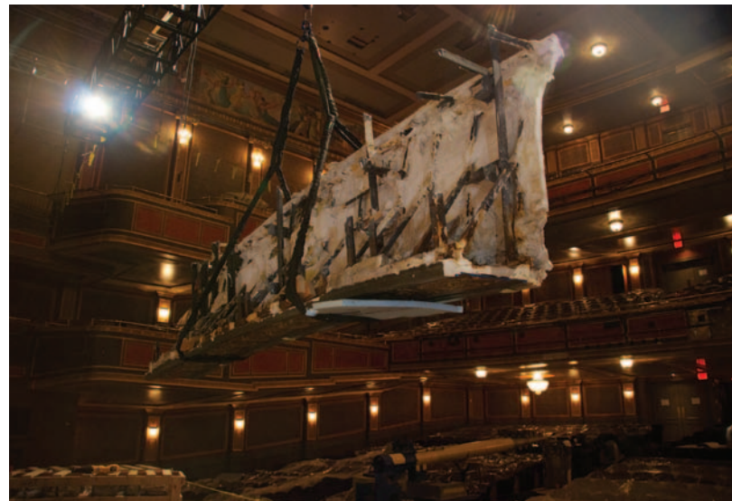
Rear view of the proscenium being raised
