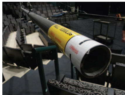
Pipe Battens at the new DePaul University Theatre School
