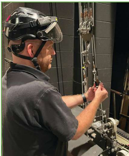
The author inspecting a swage sleeve termination with a Go-Gauge. Photo credit: Avery Spellmeyer.
