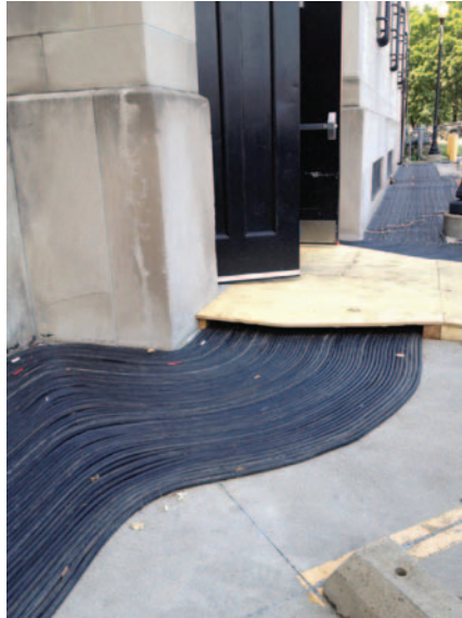
Laying a river of 4/0 cable for Jupiter Ascending
