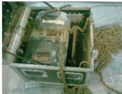
Figure 4 – An example of a worst case scenario—chain hoist that is used solely for outdoor events and is stored in a trailer between events, without preventative maintenance being completed between shows at a company shop.
