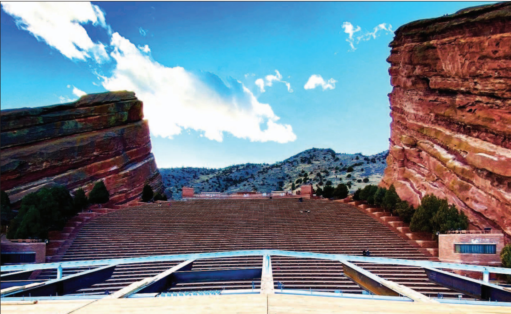
Looking from the stage roof during construction.
