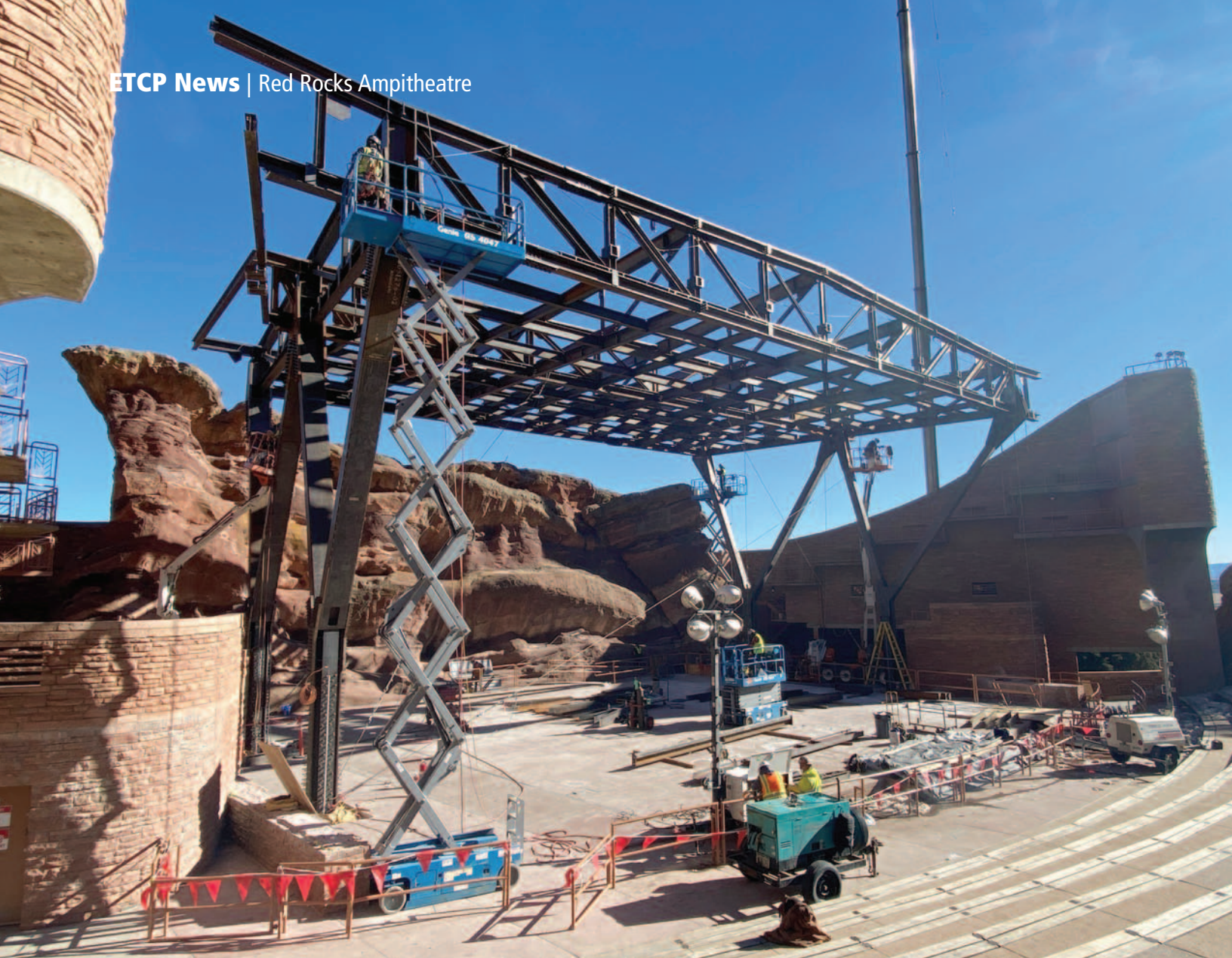
Construction of the roof structure at Red Rocks Amphitheatre.
