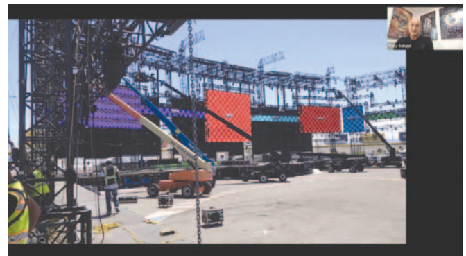
Joe Clayton shared a detailed checklist for developing his design plans to hanging today’s massive video walls—all before he leaves the office.
