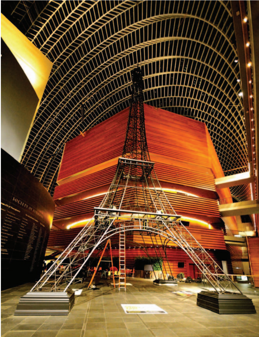
In 2012, Proof Productions, Inc. was commissioned to build an 85' tall "Eiffel Tower" scenic element, designed by Mimi Lien, for the Philadelphia International Festival of the Arts in the Grand Atrium of the Kimmel Center.
